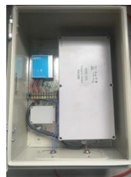
Battery and controller housed in lockable cabinet.
